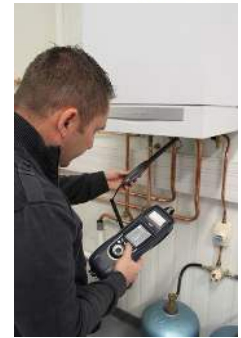
Ambient CO checking
