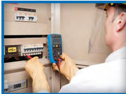
**Electrical maintenance** operations are optimized thanks to the  $V_{\text{LowZ}}$  low-impedance voltage measurement function which frees you from the effects of stray voltages linked to computer equipment or other sources when carrying out maintenance work in offices or tertiary buildings.
